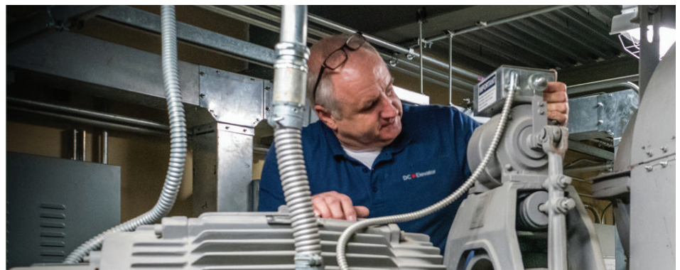
DC Elevator Technician Inspecting an Elevator Motor
